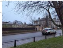
View 7 - Site photograph (2025) Existing boundary wall to New Square
