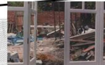
View 2 - Site photograph (c. 2000) Conservatory being built in the background
